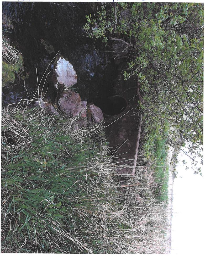
BACKSIDE OF HEADWALL, CLAY TILE IS ENCASED IN CONC
